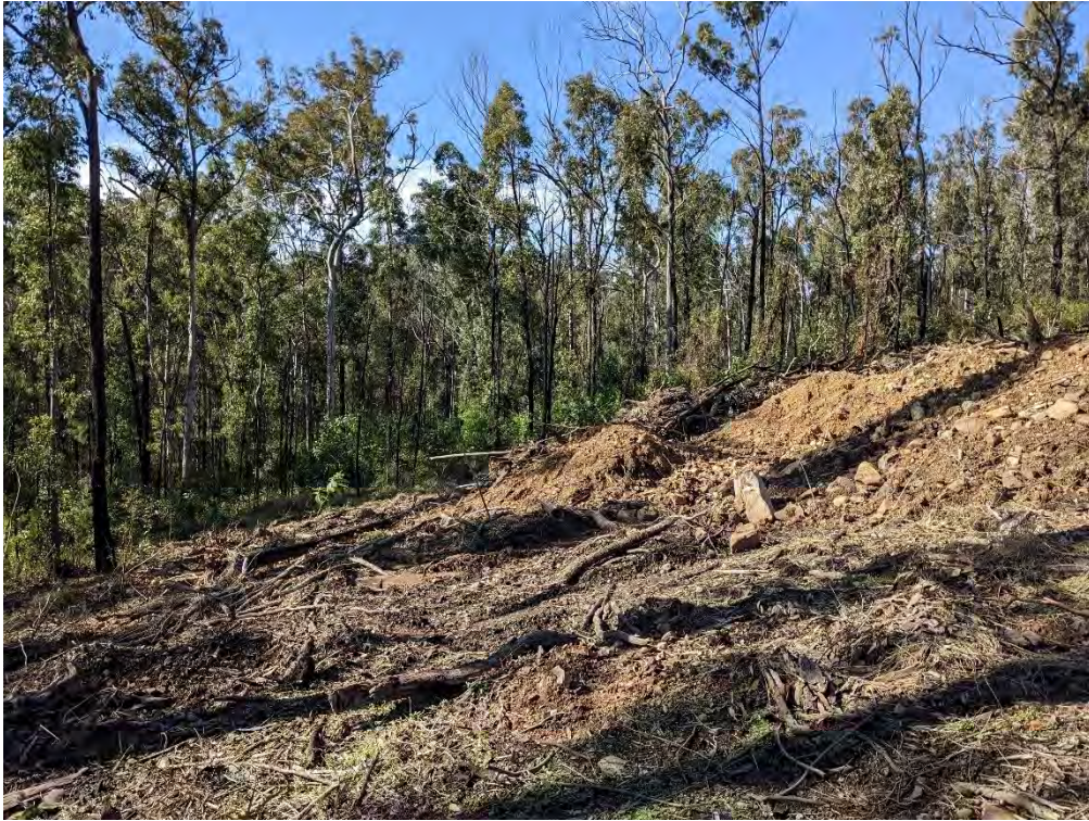
Recently cleared area to the east of the main pit
