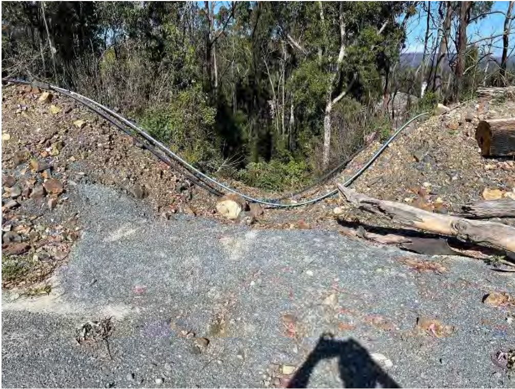
Plate 9: Drainage feature at OB3 -note the temporary bund
