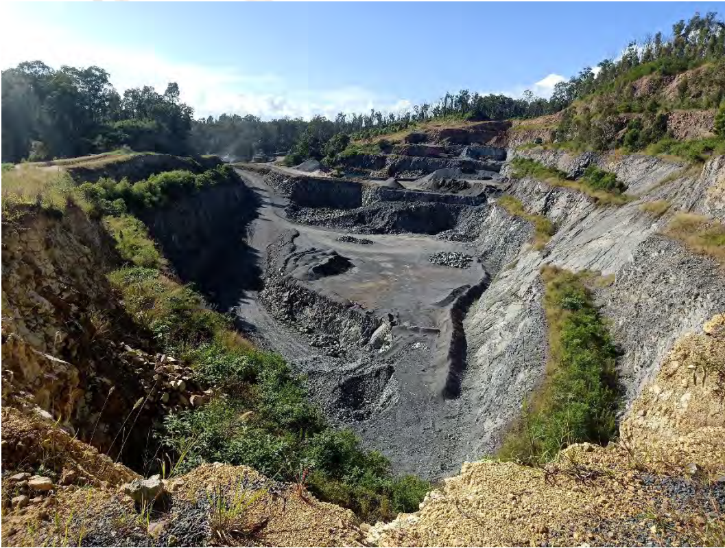
Plate 7 Rehabilitated benches along both sides of the AP benches and material falling into AP dam.
