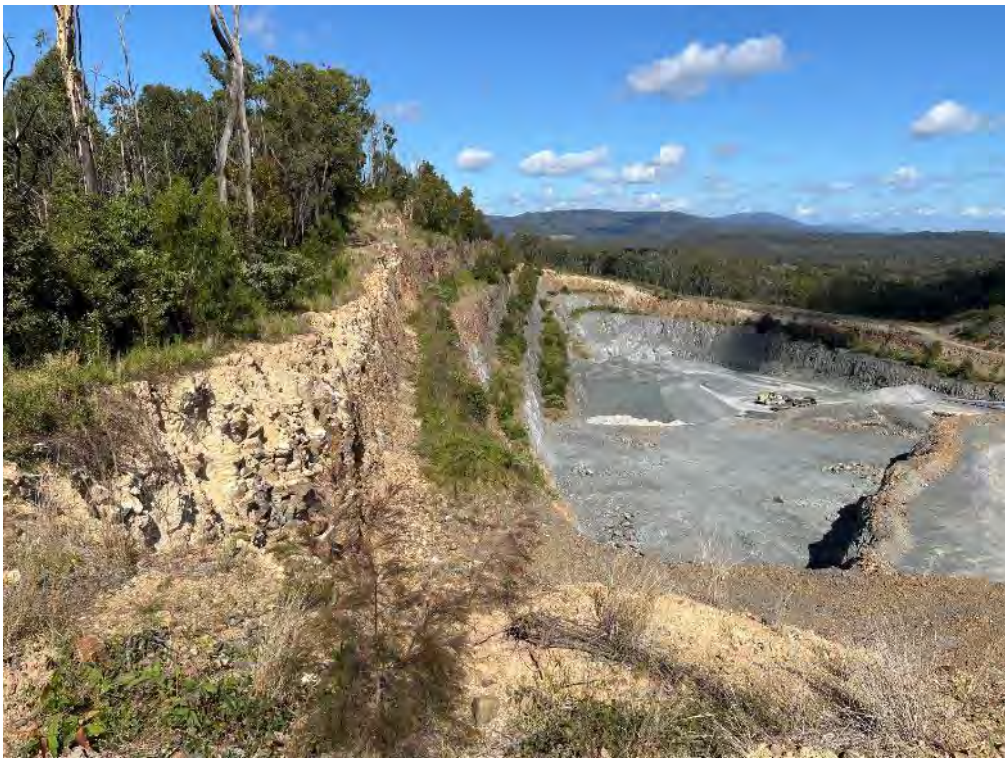
Plate 10: OB4 showing the eastern Active Pit Area Benches. Note the unstable rock face at the left and the narrow benches
