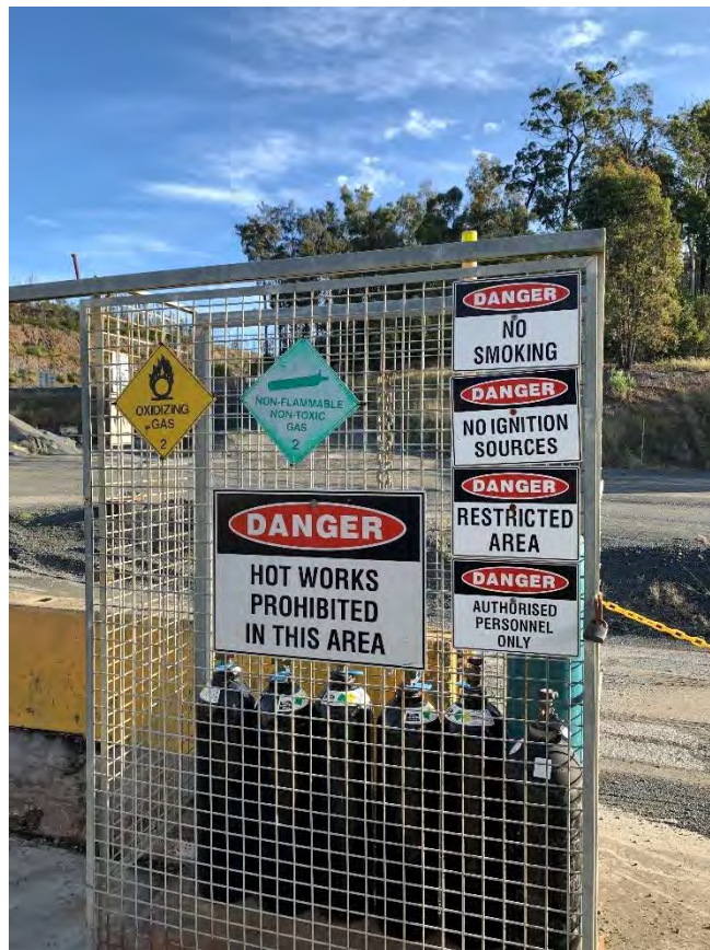
Secured dangerous goods storage on site
