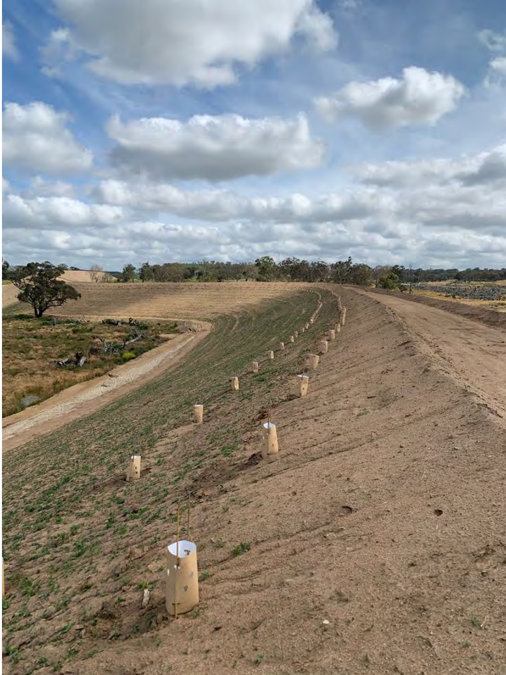
Photo 1: Grass seeding, and trees planted on the bund wall.
