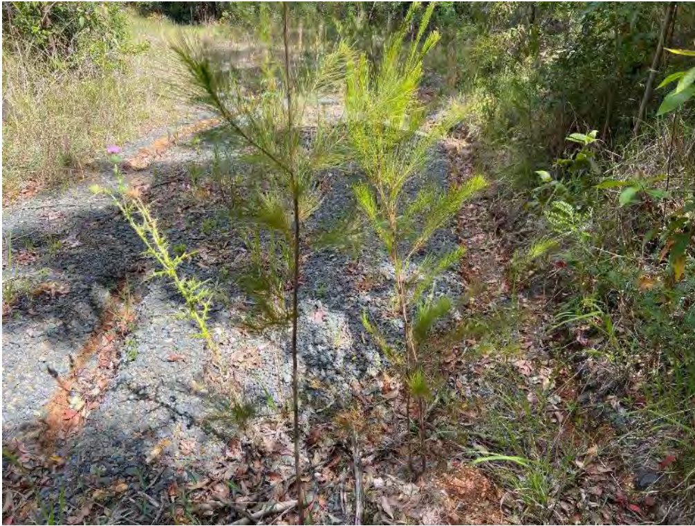
Plate 13: OB11 – rill erosion on access track (not active) in background and self-regenerating Allocasuarina spp. in foreground
