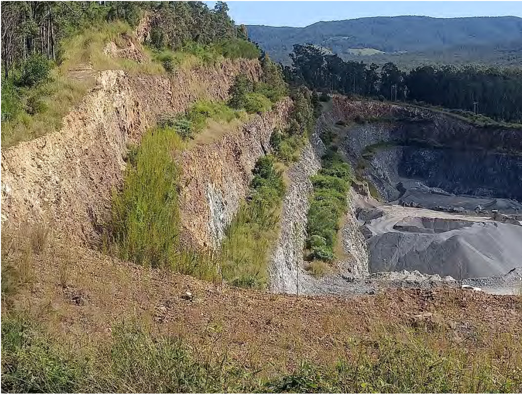
Plate 5 Rehabilitated benches along the eastern side of the AP area.
