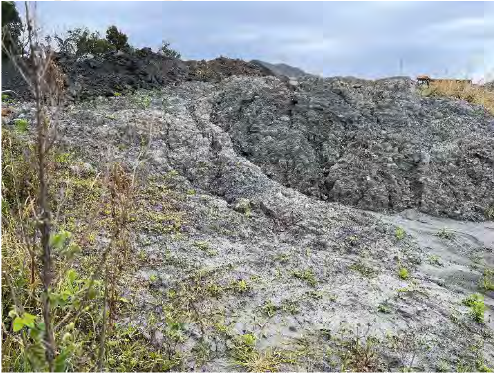
Plate 7: OB1 showing erosion of unconsolidated material on the Overburden Stockpile Area
