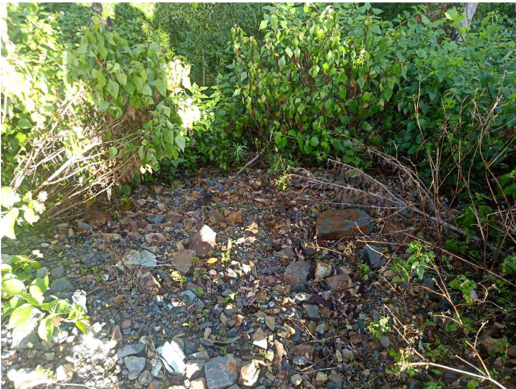
Plate 4 Exotic species growing within a constructed drainage channel.
