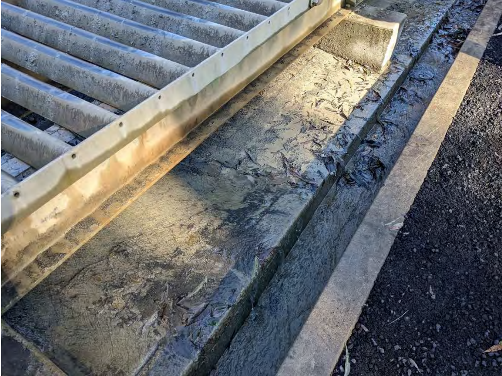
Sediment being washed from vehicle wheels prior to leaving the site.
