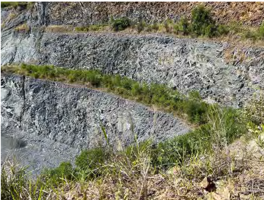
Plate 12: OB6 showing the revegetation of the southern benches in the Active Pit area. Note the lack of taller Eucalyptus species, proliferation of Acacias and exotic grasses
