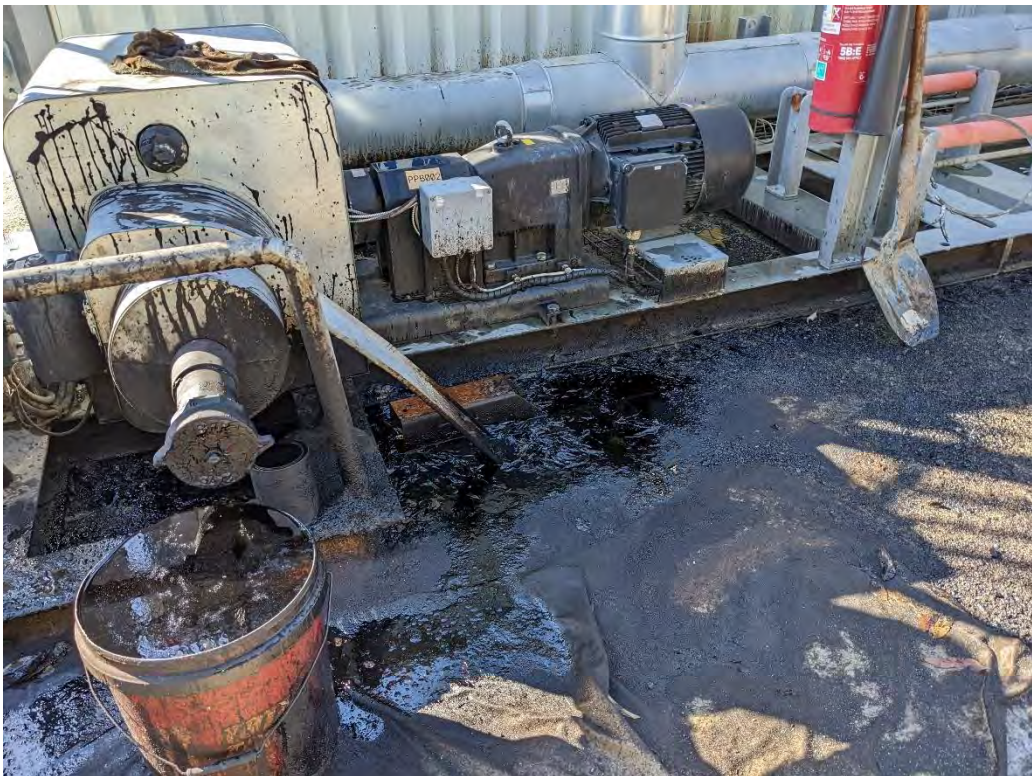
Minor hydrocarbon leakage, primarily on to geofabric, within the Downer plant area
