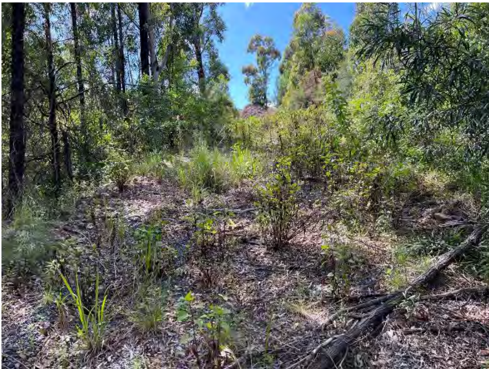
Plate 14: OB10 showing the access road to the OSA from the Settlement Dam. Minor rilling is visible bottom left, note the proliferation of weeds
