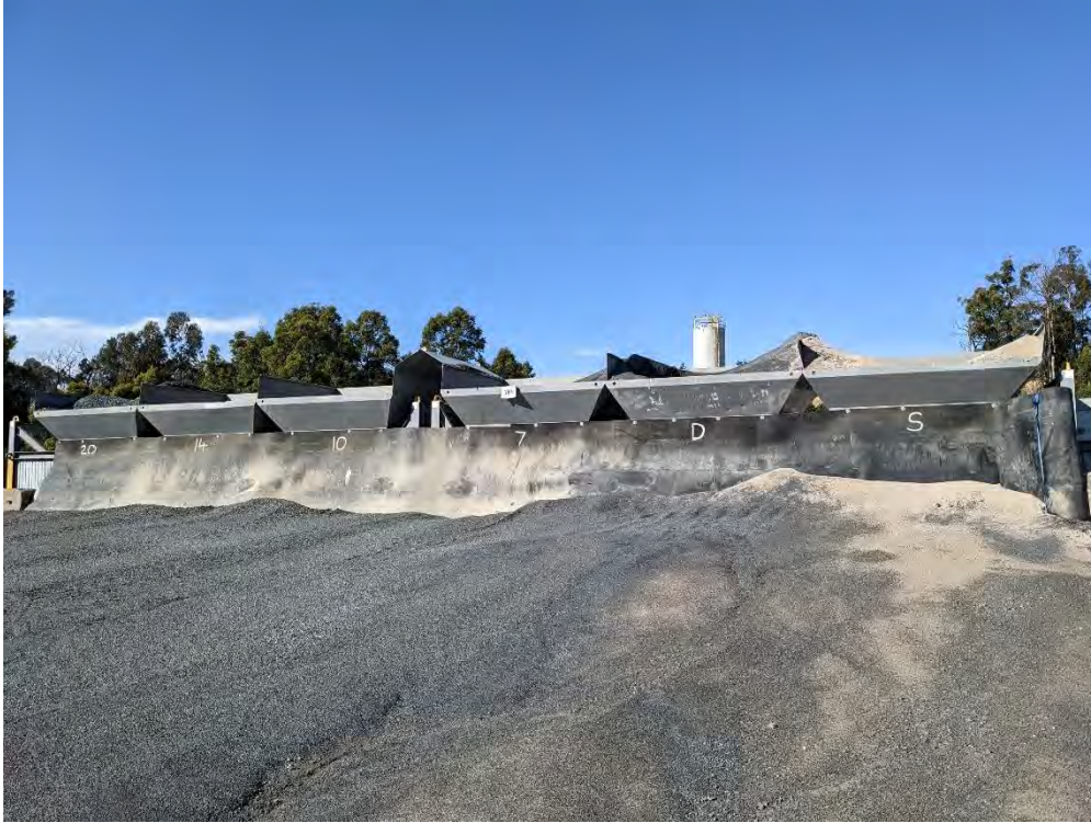
Aggregate storage within the Downer plant area, no evidence of waste asphalt being brought to the site was observed
